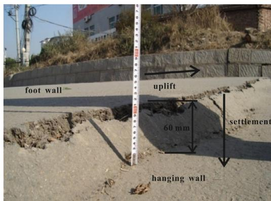
Fig. 3. Settlement of highway ramp in a ground fissure site.
